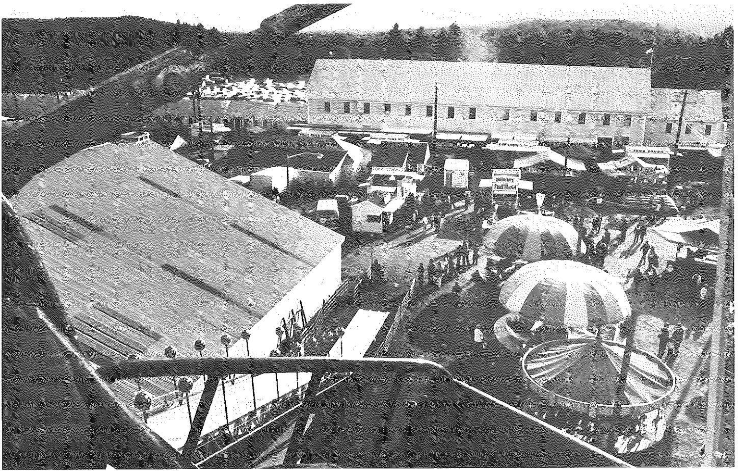
Looking at Pulling Ring, left, and Exhibition Building, center, 1960's.
